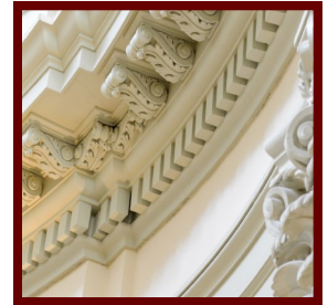
Interior of the State Capitol dome
