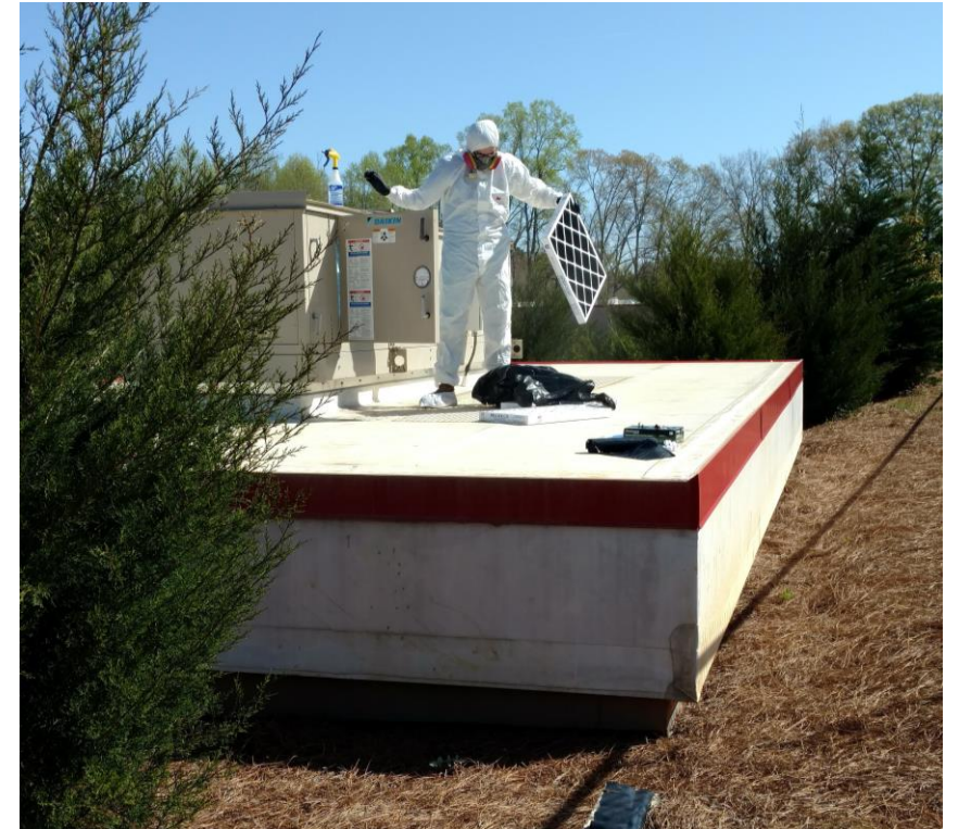
Image of Employee Changing Filters Coated in Lead Dust from Shooting Range
